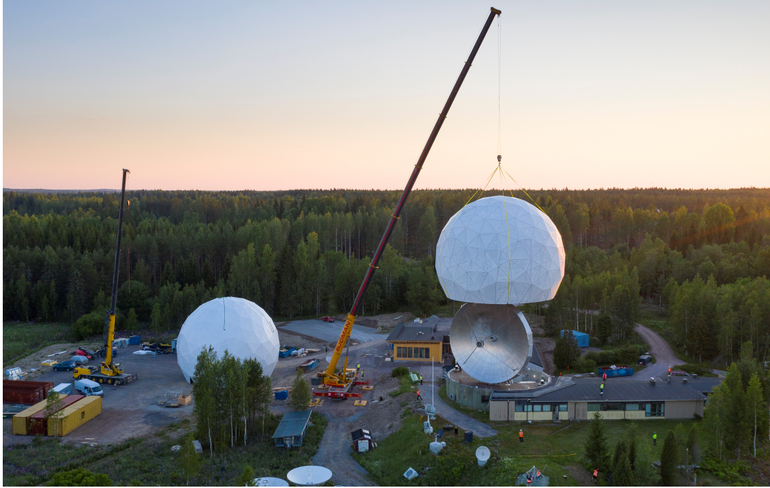
Figure 6.7: Replacement of the 14m radio telescope radome at Metsähovi.
