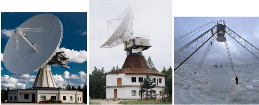
**Figure 5.11:** Left panel: Irbene Ir - RT-32 radio telescope; middle panel: Irbene Ib - RT-16 radio telescope; right: New vertex cabin mounted at the radio telescope RT-32 secondary focus.
