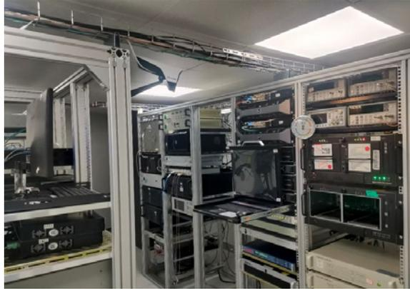
**Figure 5.14:** The digital backend systems for VLBI and single dish operations working in the walk-in electromagnetic shielding box under the telescope base.
