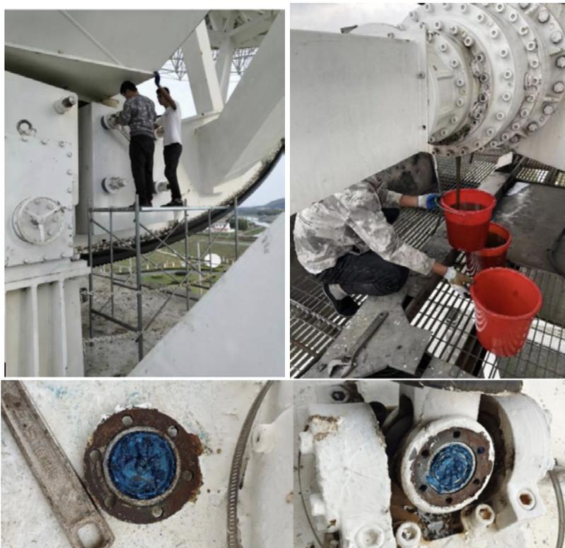
**Figure 5.9:** Maintenance of the TianMa 65 m radio telescope: top left, replacing screw spacer; top right, replacing of gear oil; bottom: checking grease status
