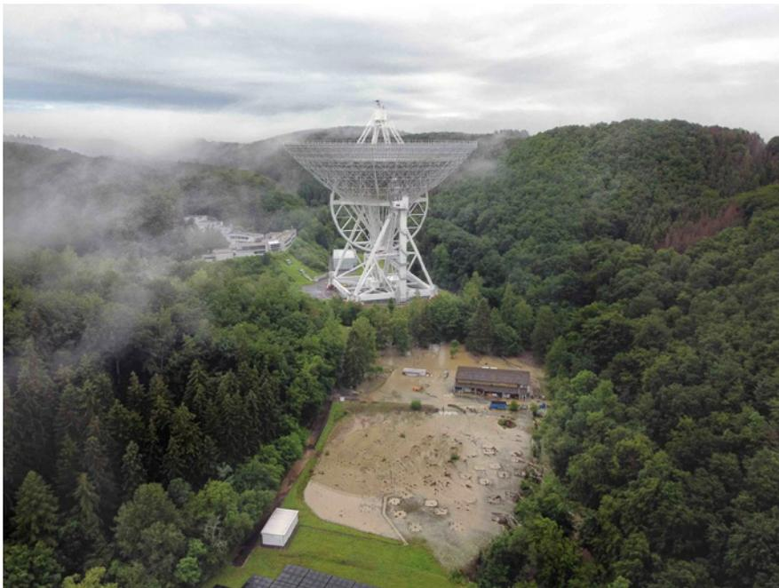
**Figure 5.8:** Aerial view of the Effelsberg radio observatory on the morning of July 15, 2021. The image shows in the foreground the completely flooded "low-band" part of the Effelsberg station of the European LOFAR telescope network. In the background the 100 m radio telescope and to the left the observatory building with control room (photo N. Tacke, MPIfR).
