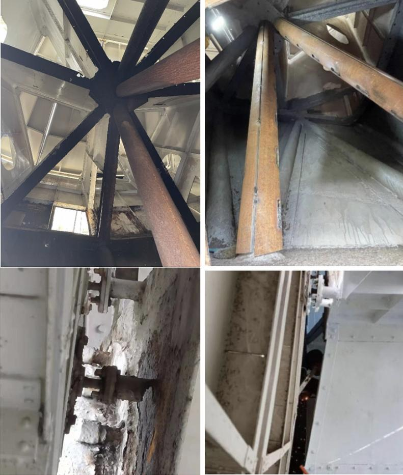
**Figure 5.10:** Maintenance of the Sheshan 25 m radio telescope: (top) structure reinforcement; (bottom) replacement of supporting bars.
